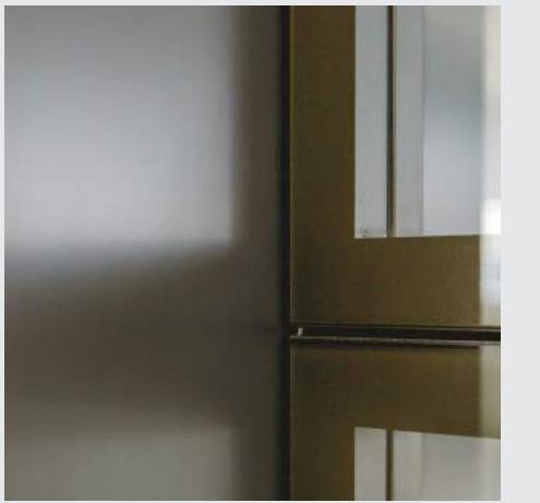
Joint of structured glass panels to a cupboard.
